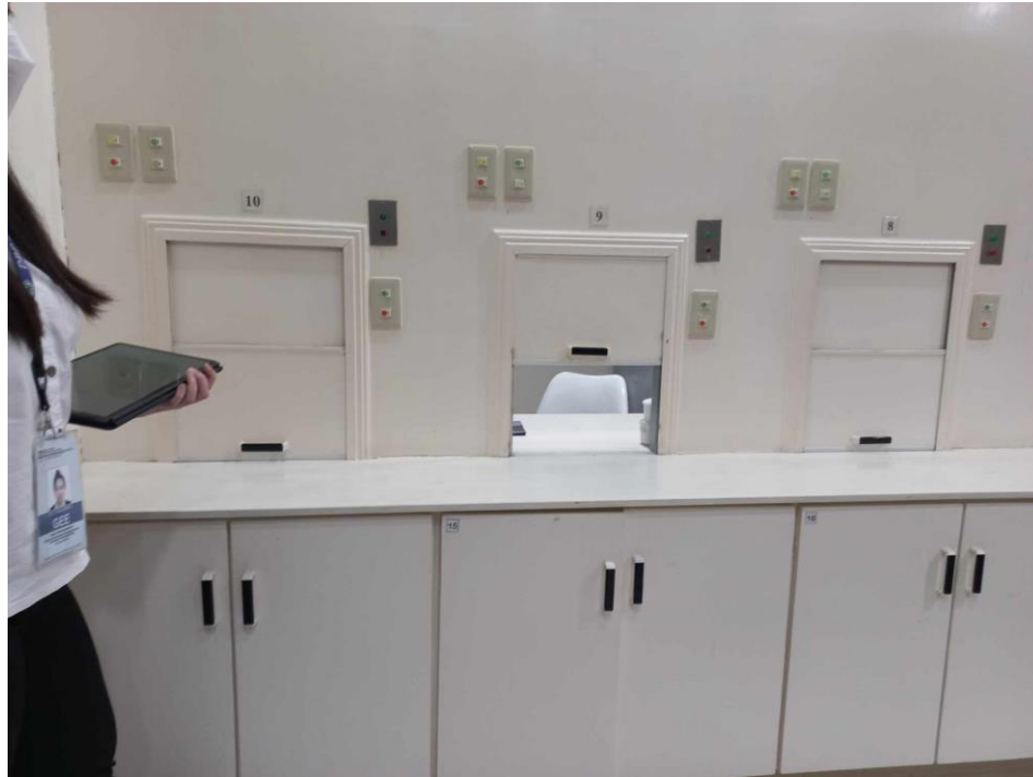
Back side of the pass-through door (Reference: DOST-FNRI)
