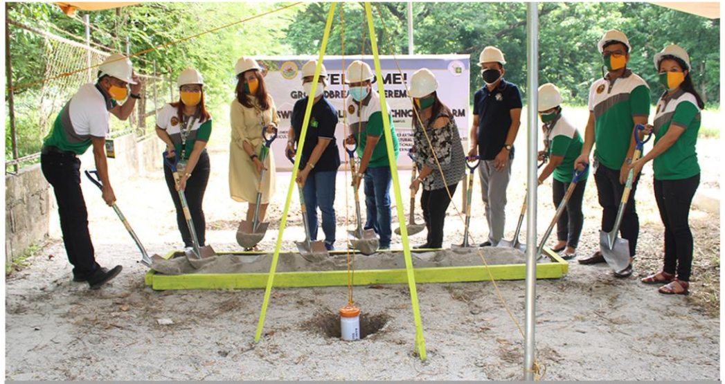
BASC officials led by Dr. Jameson H. Tan together with the DA-ATI representative during the groundbreaking ceremony.
